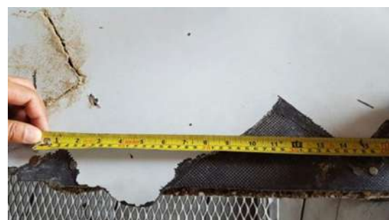
Spacing of fasteners on the debris
